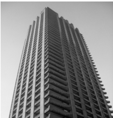
Barbican Centre Residential Tower
